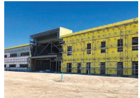
Construction continues on the new Cristo Rey St. Viator College Preparatory High School.
